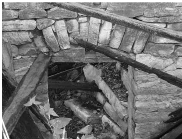
Figure 17. South end view of Kieffer 2 cave, showing arch over entrance doorway below stone house.
