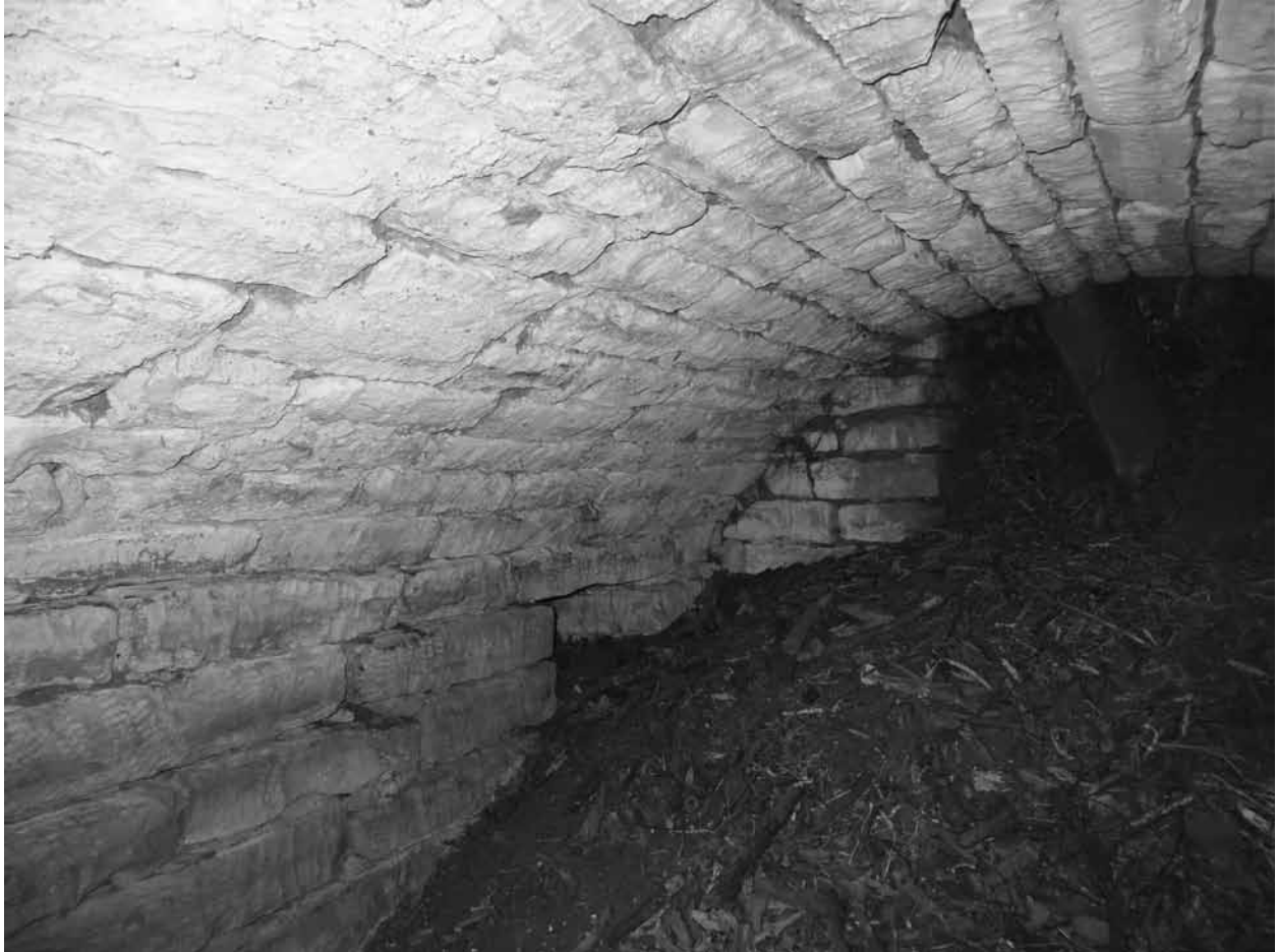
Figure 39. Northwest view of Krob cave, showing arch stones overlapping end wall, small side wall niche, and chute-type vent.
