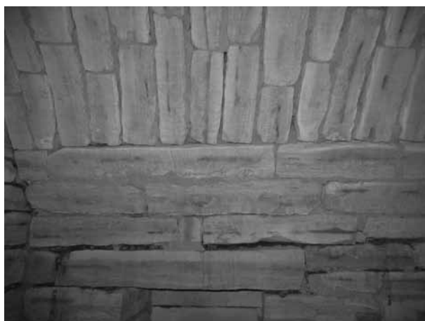
Figure 21a. East wall detail of Kieffer 3 cave, showing tilted position of topmost wall stones to begin arch.
