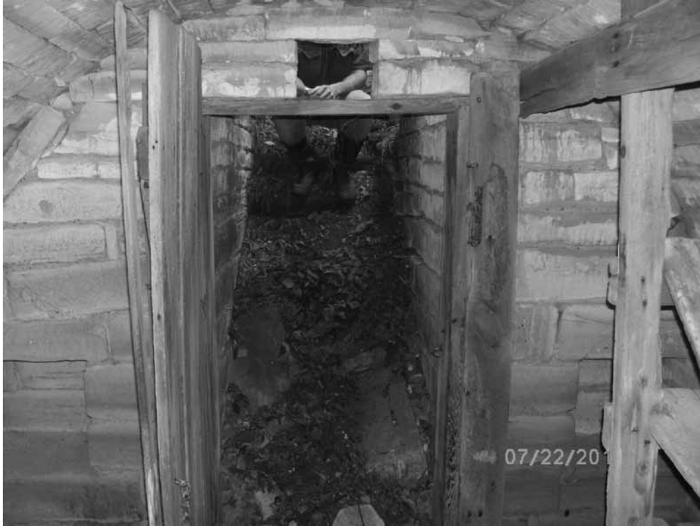
Figure 7. East end view of Filipi-Kiperta cave, showing door, window above door, and remnant of shelving.
