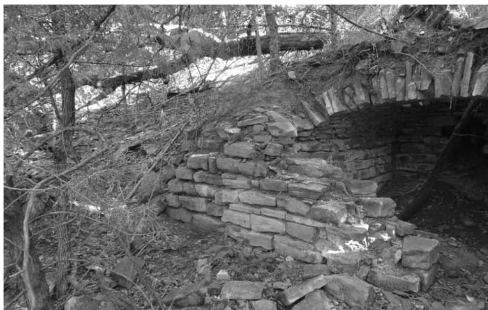
Figure 37a. Double-faced walls with rubble cores. Southeast view of Hubbell cave north wall.
