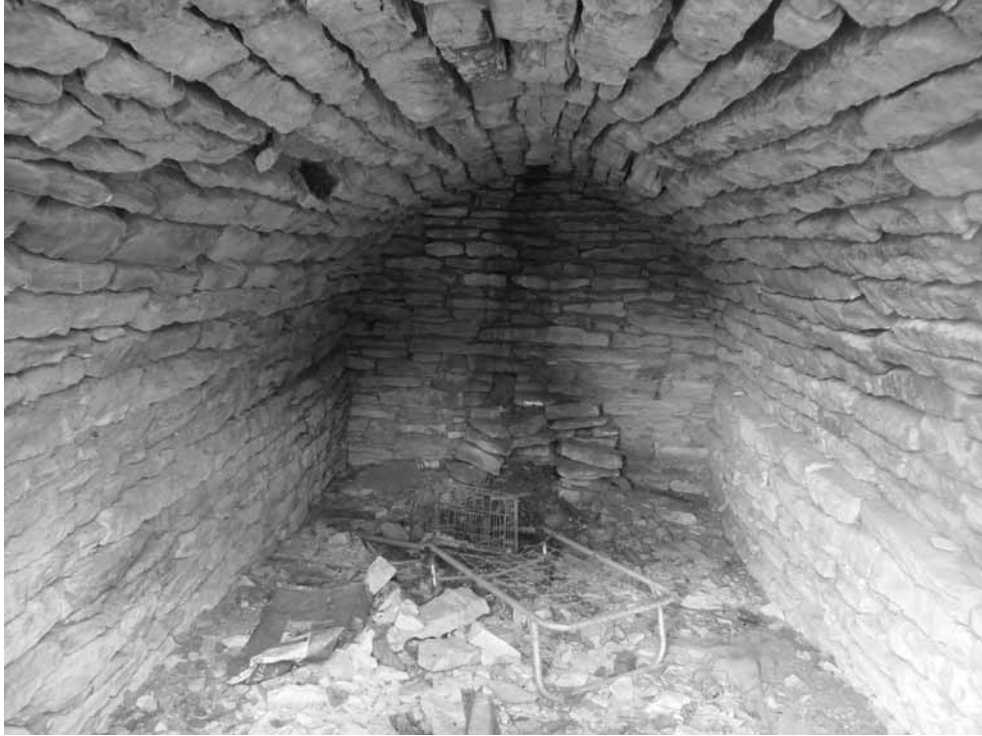
Figure 22a. West wall view of Wagner cave, showing ceiling construction and firebox against wall. Note narrow shelf on north (right) wall at base of arch.
