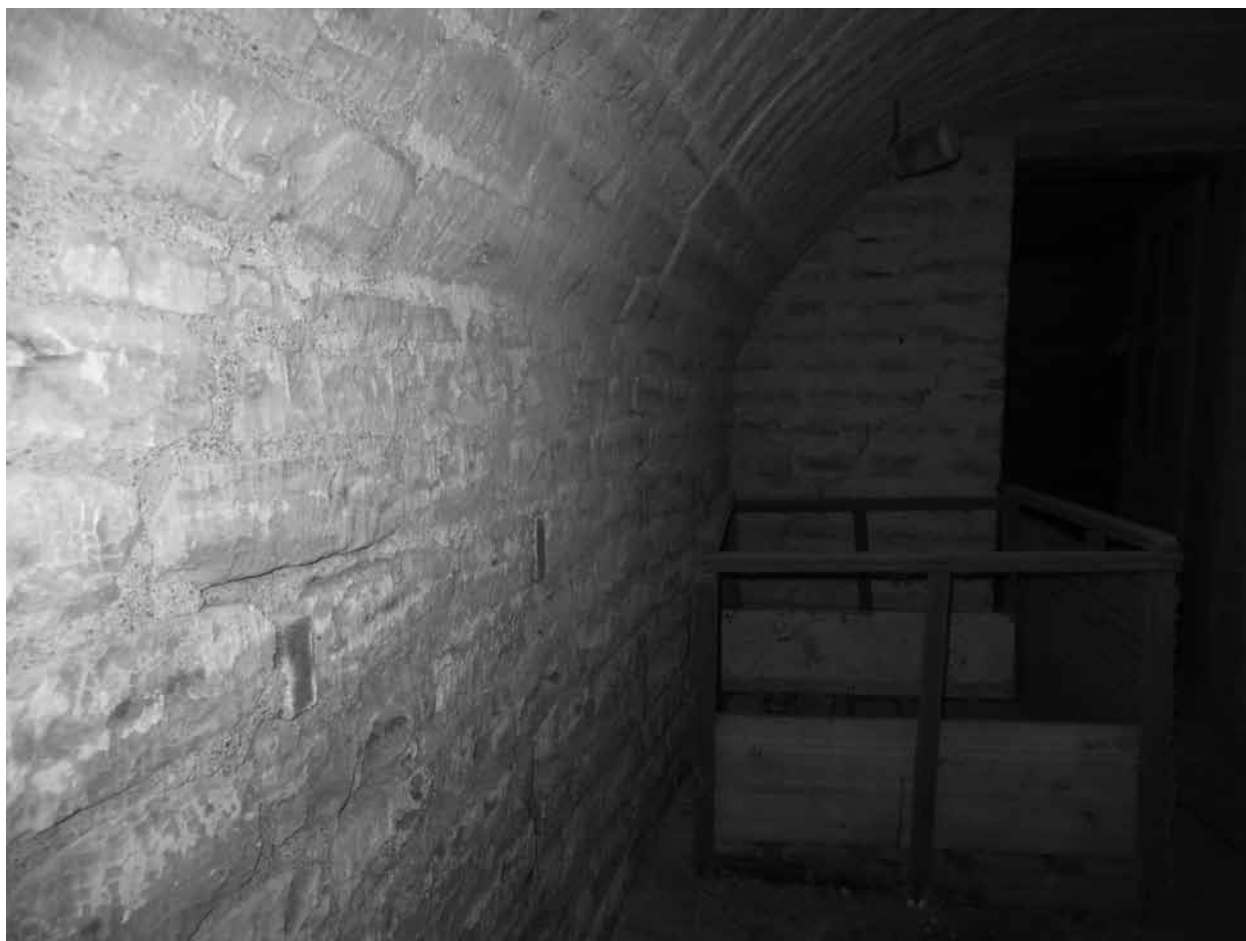
Figure 10. North wall view of Shimek cave 1, showing top wall stones tapered inward to begin arch.
