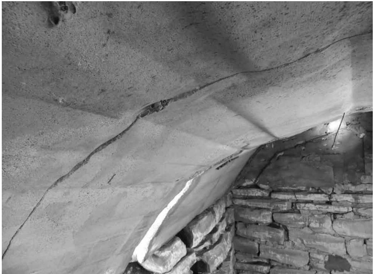
Figure 13. Concrete arched ceiling of Tietjen cave with board impressions.
