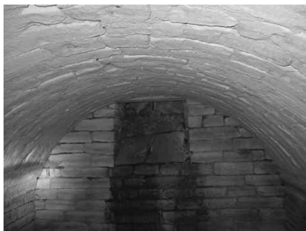
Figure 21b. South wall view of Kieffer 3 cave, showing tilted position of topmost wall stones to begin arch and chute-type vent.
