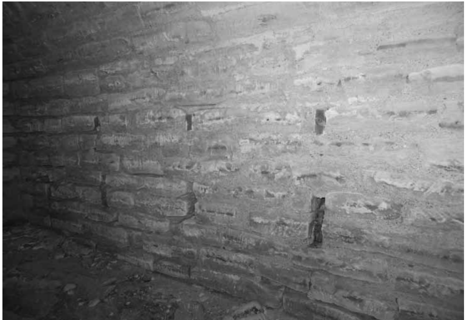
Figure 11. North wall view of Shimek cave 1, showing wooden blocks set in wall as shelf attachments.
