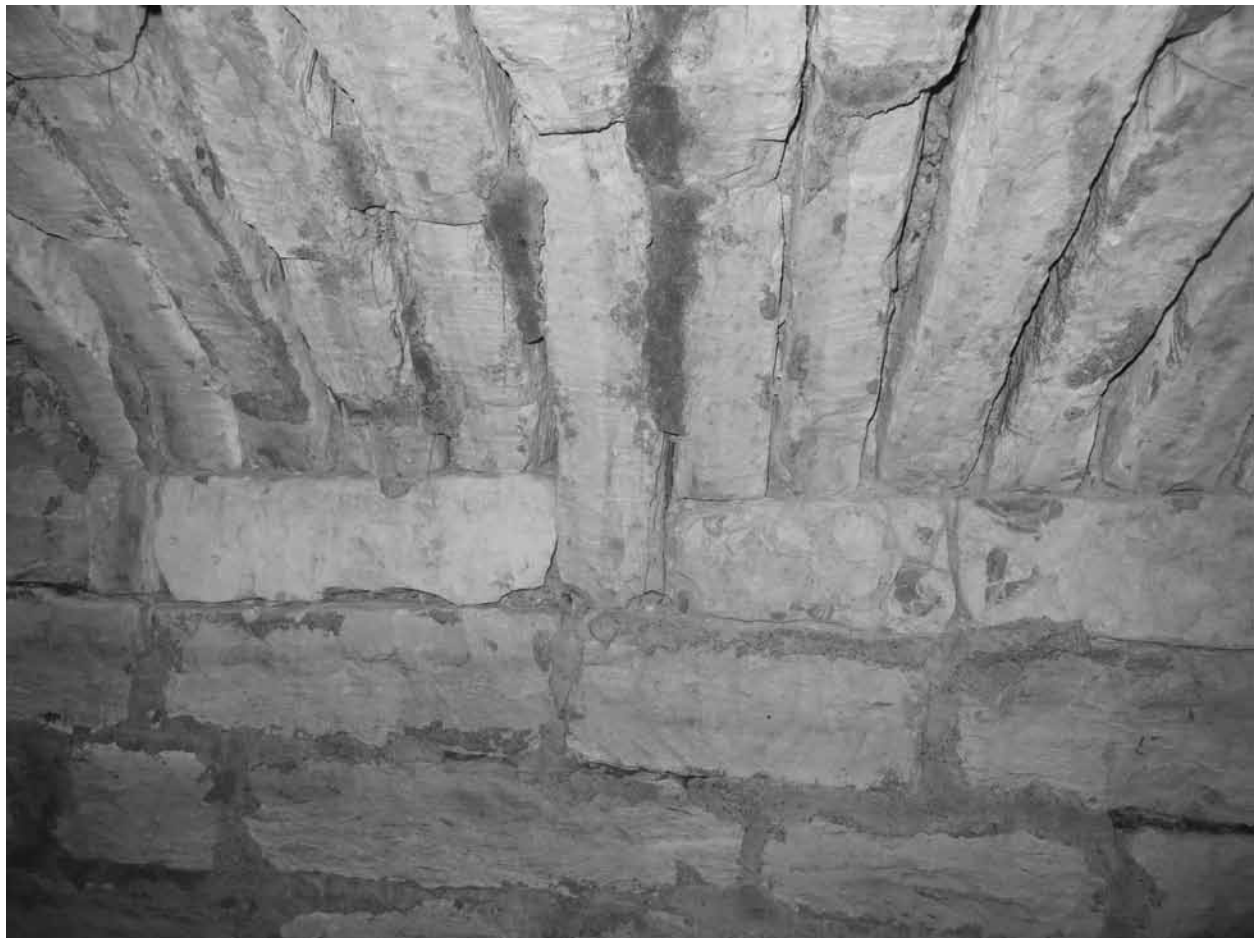
Figure 31. South wall detail of Lojka-Svojgr cave, showing arch stone interlocked with top wall stones.
