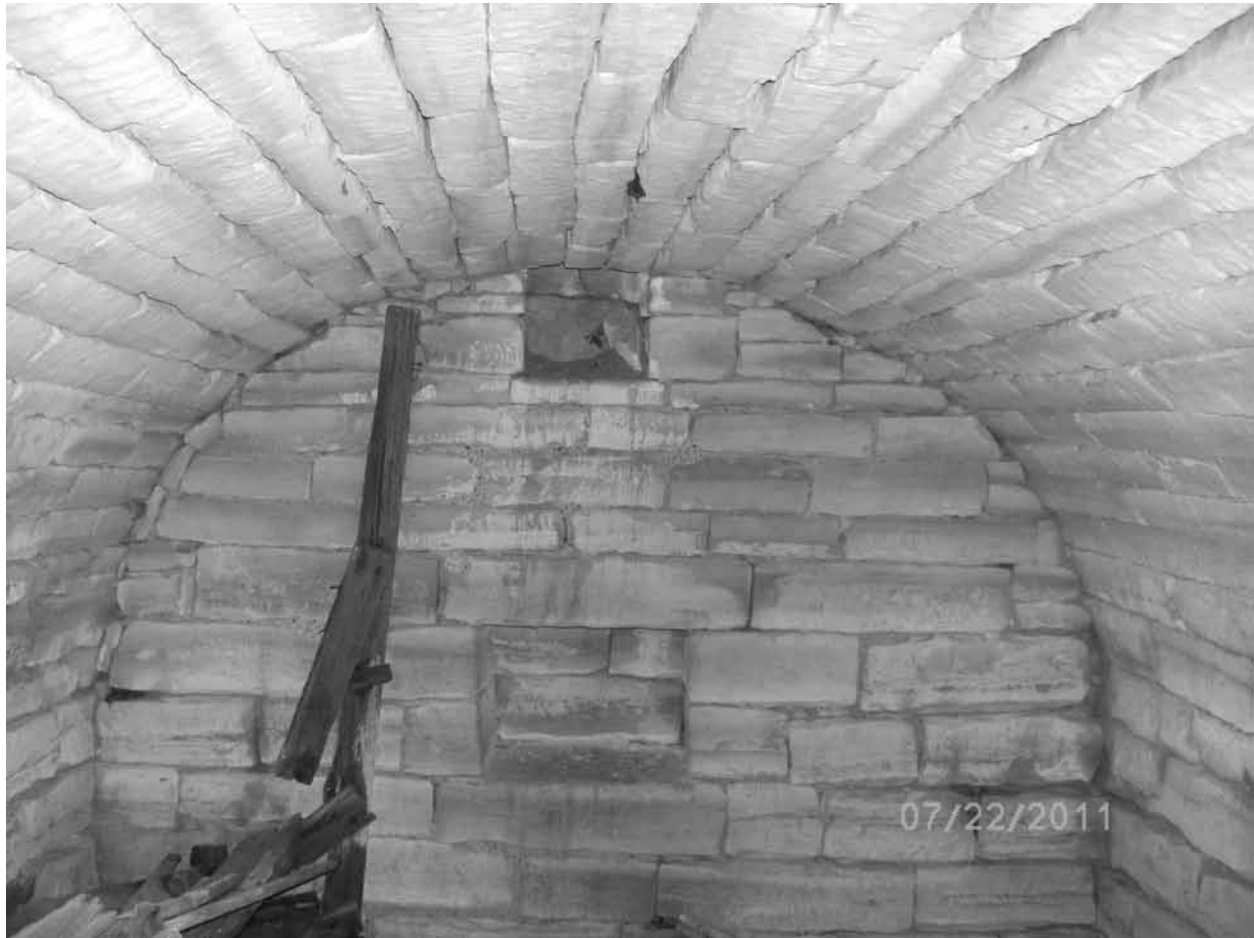
Figure 6. West end view of Filipi-Kiperta cave, showing niche, vent, and arch stones overlapping end wall.
