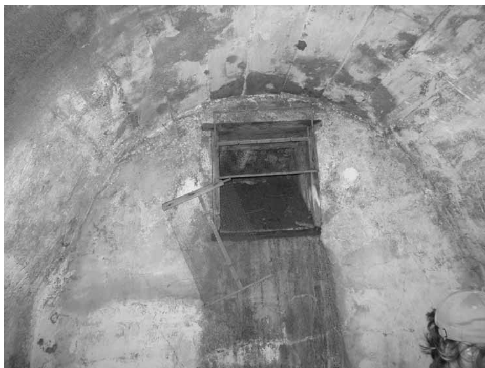
Figure 16. Ceiling and south wall view of Jehlik cave, showing chute-type vent and board impressions on ceiling.
