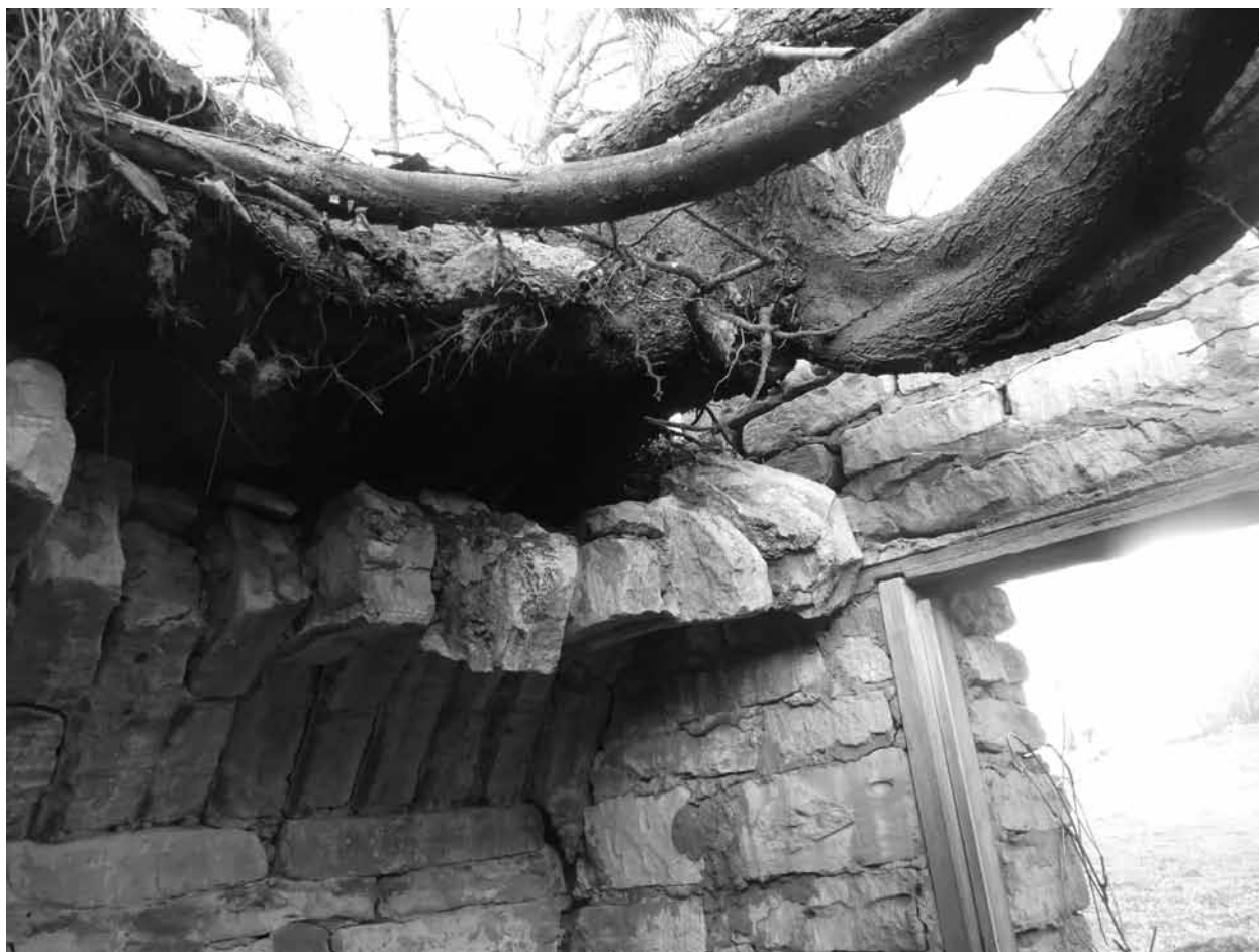
Figure 29. View of Lojka-Tuma cave, showing perpendicular arch stones and partially collapsed ceiling due to tree roots.
