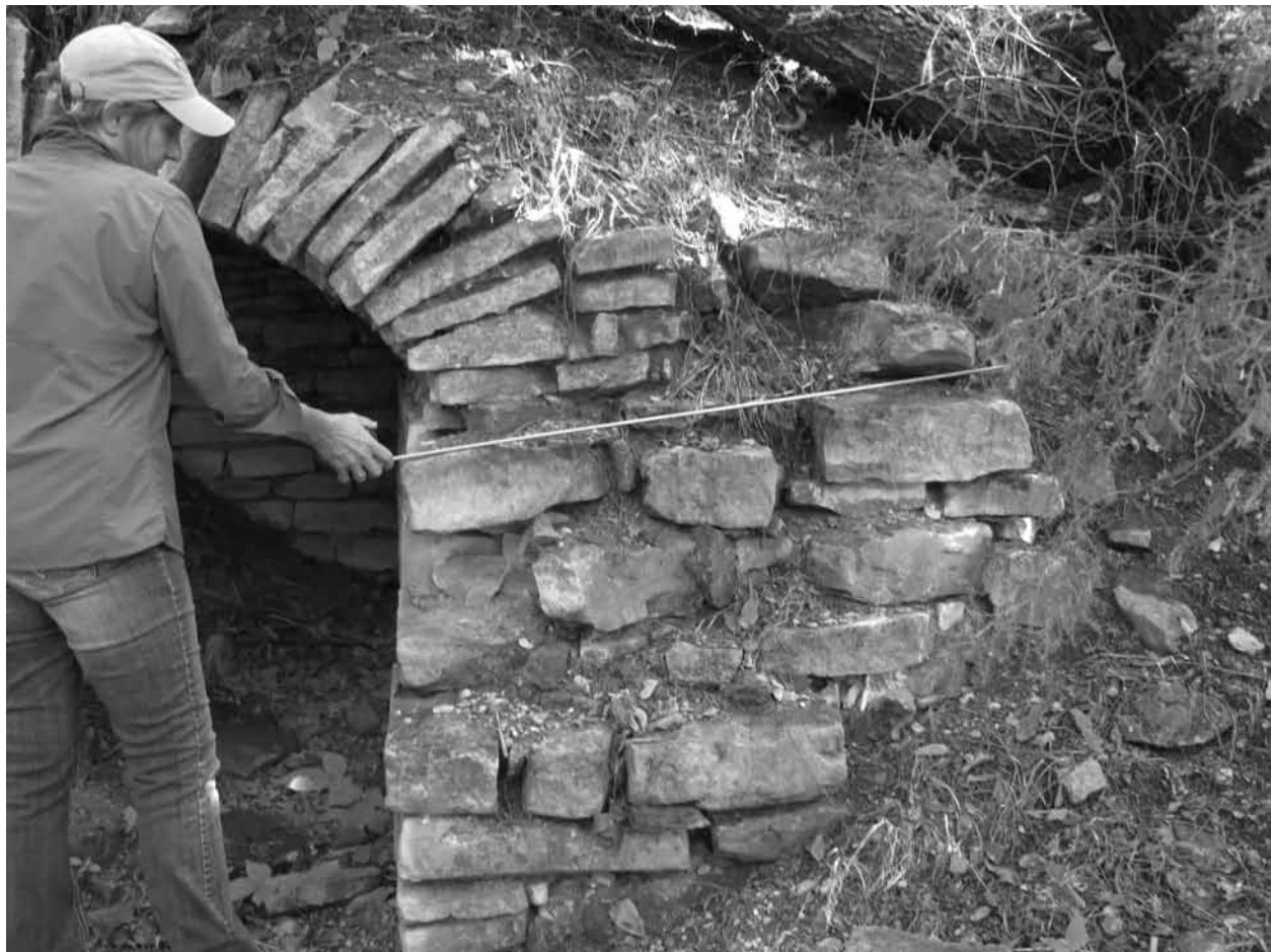
Figure 14. South view of Hubbell cave, showing buttressed end of west wall and door opening.
